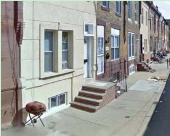
The brick stoop does not maintain the same stoop orientation that has been established on this street.
