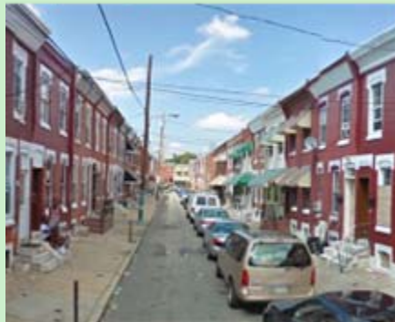
1545 Garnet Street | View: North
