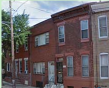
2240 Reed Street | View: South
