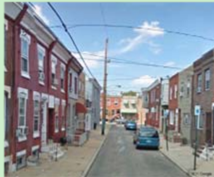
1519 Garnet Street | View: North
