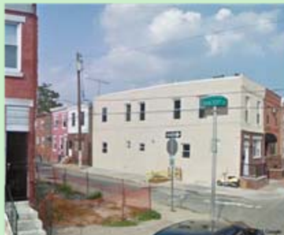
1621 Reed Street | View: North-East
