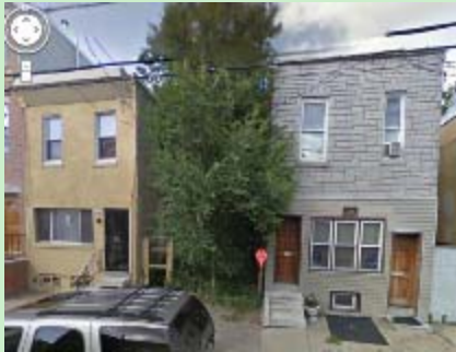
These homes use stucco, vinyl and simulated stone veneer. Materials that are not characteristic of the Point Breeze neighborhood.
