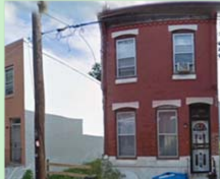
2212 Reed Street | View: South
