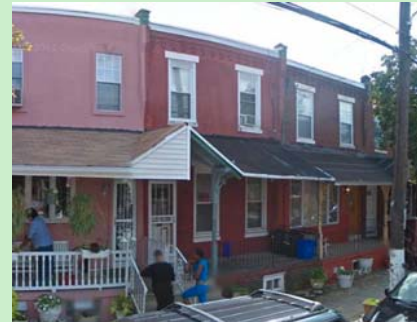
The left porch does not maintain similar styles or materials to the original porches on this block.
