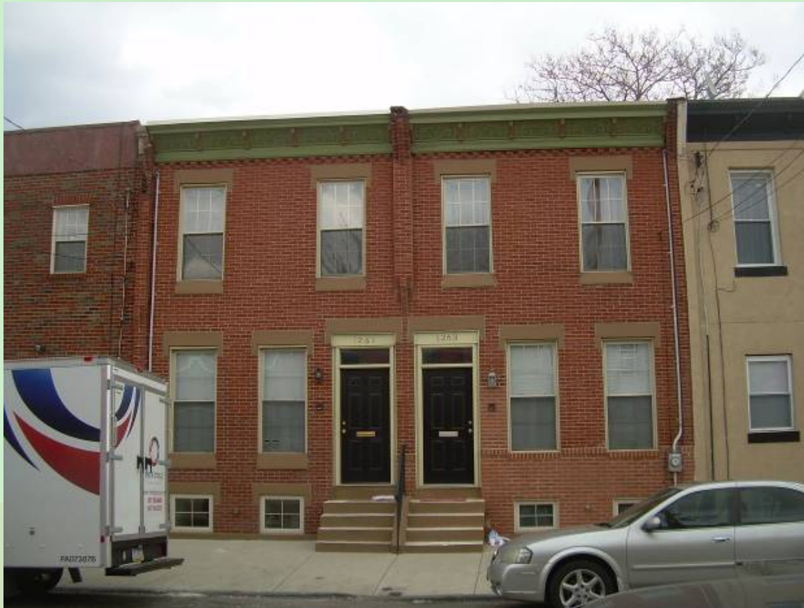
Newly constructed houses on the 1300 block of 22nd St.
